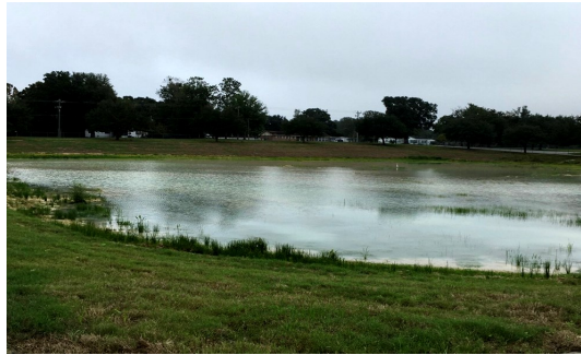
› Drainage project on Troy Road
