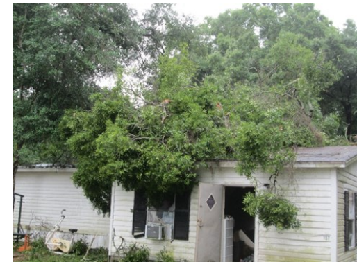
› Good Friday storm damage
